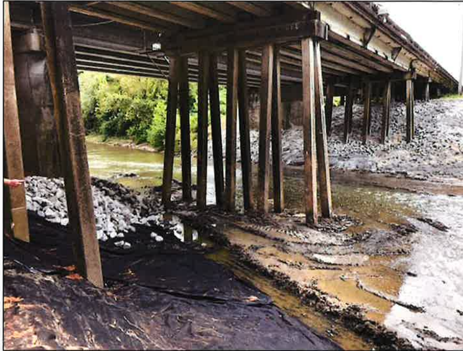
Bridge Piers after Rip Rap and Grouting to prevent erosion in the future
